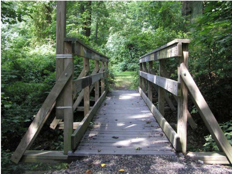
Pedestrian Footbridge, Borough Park
